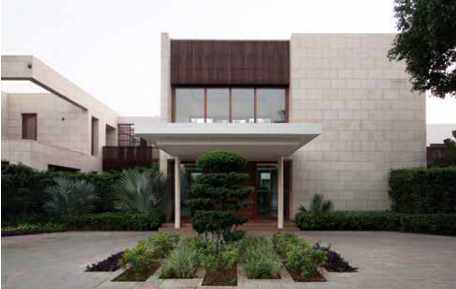
House of Bridges, New Delhi
